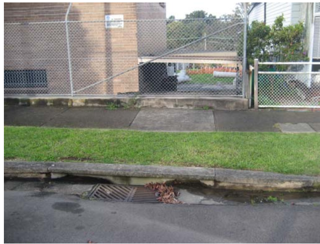
Figure 1: View from Edna Street along western site boundary showing kerb inlet pit at the depression.
