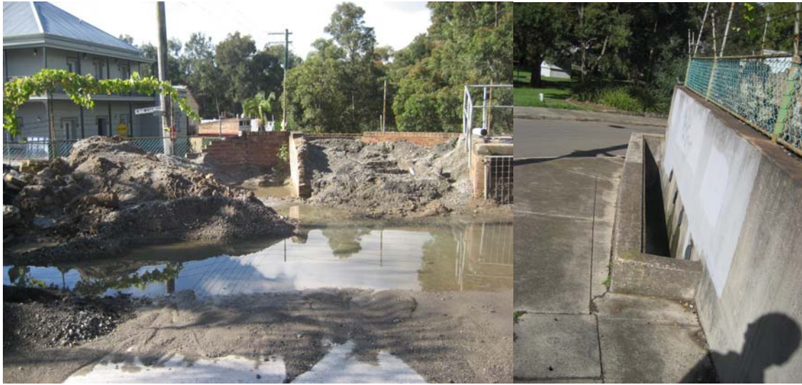
Figure 2: Left shows ponding of overland flow on the north-east point of site; right shows the stormwater drainage structure on the corner of Piper and White Street.
